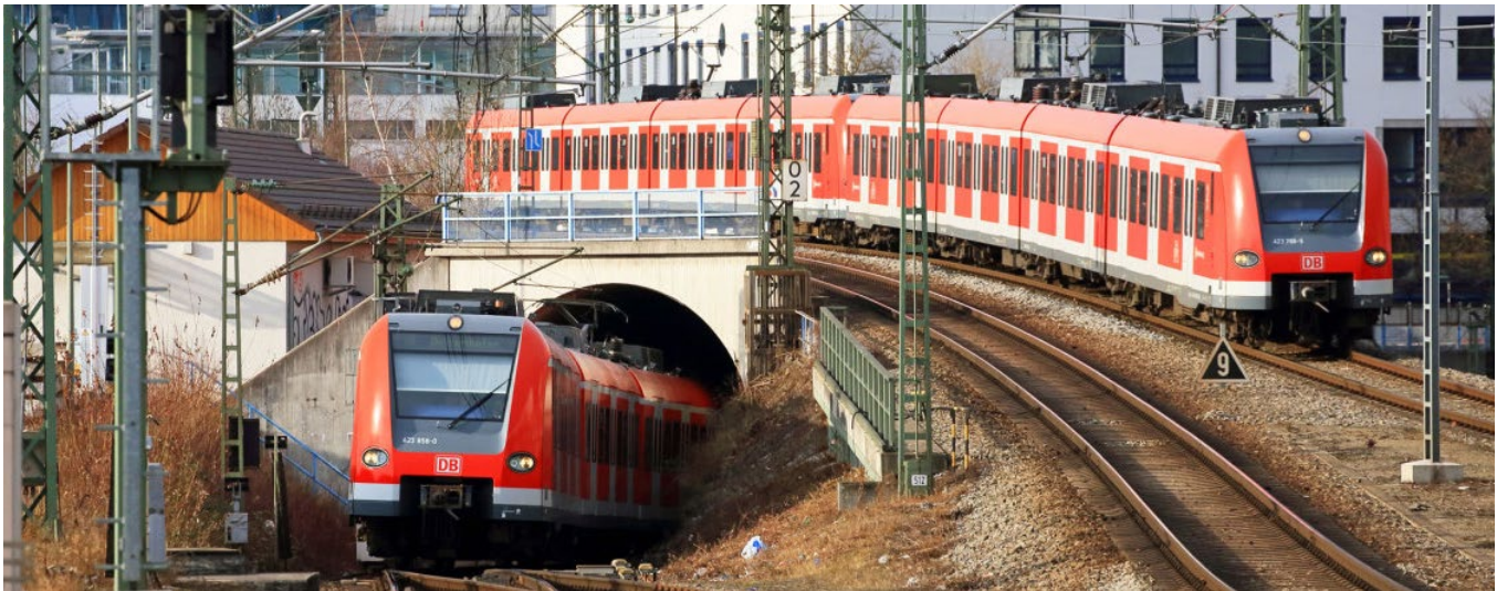
This flyover in Germany illustrates how much smaller grade separations can be with modern trains. (Image: Deutsche Bahn)
